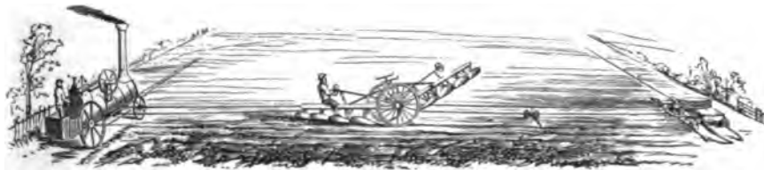
Fig. 8.—Fowler's Anchor, Engine, and Plough at work.
